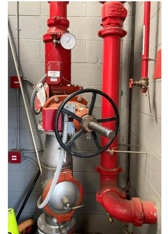
Figure 6: Fire Riser
